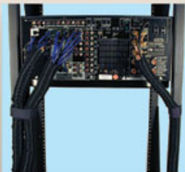
Typical Rack Install
