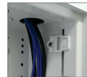
Installed SMC for affixing sidewall to stud.
