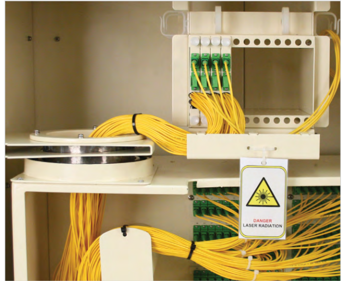
Fiber Management and Bend Radius Control
