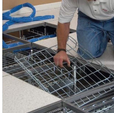
Place 2' tray sections in position.
