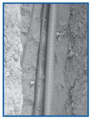
Lay conduit in the trench as straight as possible. Avoid undulations up and down and side to side.
