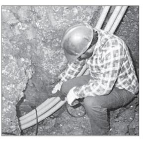
When soil conditions do not permit direct burial of cable, use Carlon P&C Flex<sup>®</sup> Nonmetallic Corrugated Conduit to protect the cable. A lower coefficient of friction provides easy wire pulls on location. flexibility eliminates the need for elbows.
