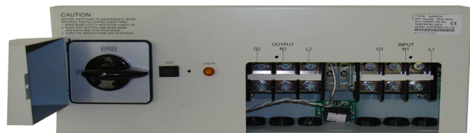
Maintenance Bypass Switch with covers off
