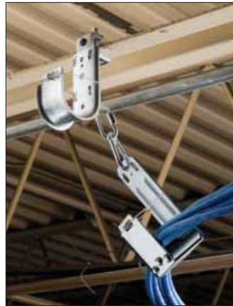
CATHPLR cable puller assembly
