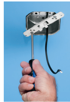
1 Attach SC5 bracket to box.
