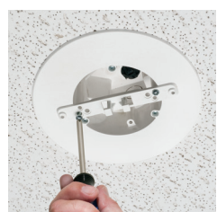
5 Install mounting bracket to inside of box.
