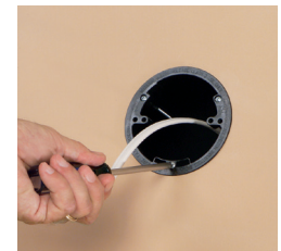
2 Pull cable and tighten mounting wing screws to hold bracket secure.
