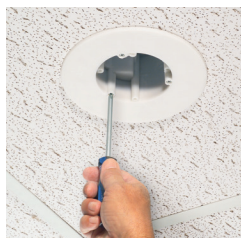
2 Align box as necessary. Tighten mounting wing screws.
