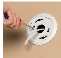
3 Install mounting plate per manufacturer's instructions.
