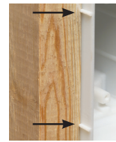
Positioning tabs for new work
