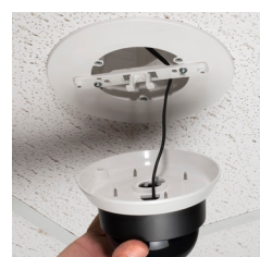
6 Mount camera to mounting plate. Place assembly on bracket. Turn clockwise to lock. Install set screw.
