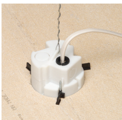
4 Install supplied NM94 cable connector (1/2" or 3/4").
