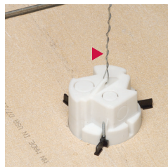
3 Wrap drop wire twice through loop on top of box and around a framing member above ceiling. Wrap wire around itself six times minimum in both instances.
